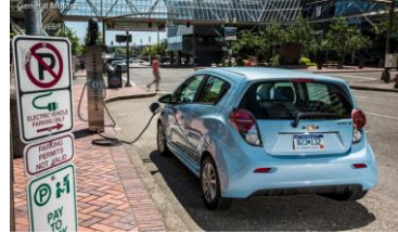
Fig. 4. Electrical vehicle charging station in a city. https://cdn.autocentre.ua/images/stories/2014/10/08/b/genera-l-motors-planiruet-rasshirit-lineyku-eko-modeley-4.jpg
